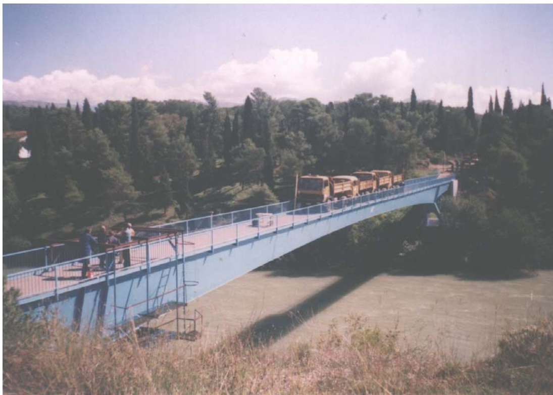
Picture 1. Position of the proof load during the structural testing
